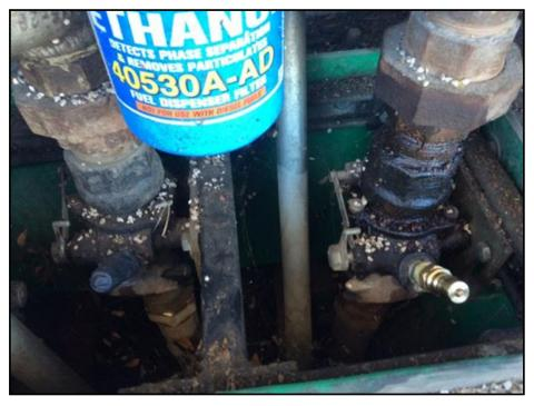
**ANSWER**: The test valve/port is below the shear/shut-off valve; therefore, if it breaks off it will render the shut-off valve useless. To correct this issue, take off the 2" test valve/port and install a plug.
